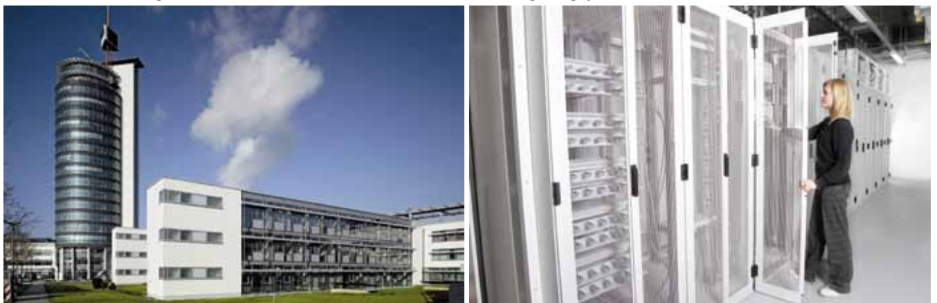
Photos below from left to right: TDS tower on Firmesitz in Neckarsulm, IT cabinets, fire extinguishing system and server cell in the TDS data center Quelle: TDS AG
